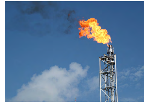
The lack of suitable natural gas infrastructure has raised prices and pollution by forcing reliance on higher-cost resources, such as oil-fired power plants.
