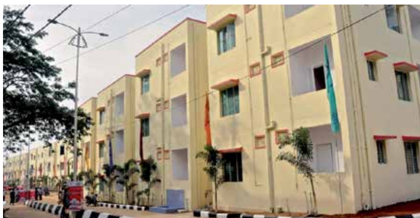
Figure 2 Newly constructed residential towers at the IDH Colony, New Bhoiguda, Hyderabad, commissioned in November 2015.
