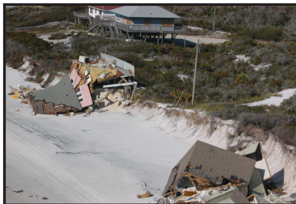
Damage was widespread on St. George Island after Hurricane Dennis in 2005. (Aerial photo by Tom Meares)
